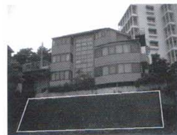
③補修工事前
