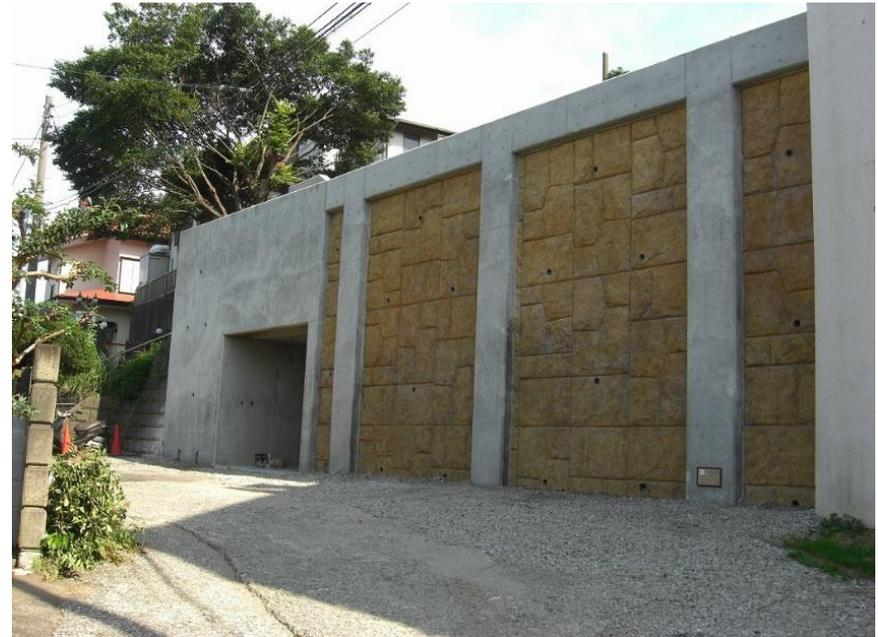
Retaining wall with small steel pile constructed by pre-bored method
