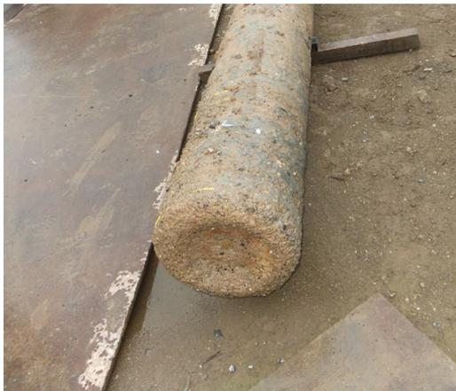
Fig. 12 Pile tip situation (S-Pile)
